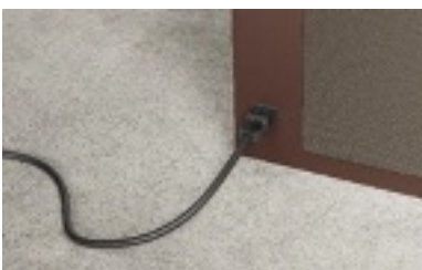
Illustration 3 - Power and data connection through column side
